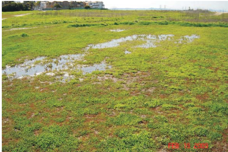
Ponding clearly evident at Fairview Park.
