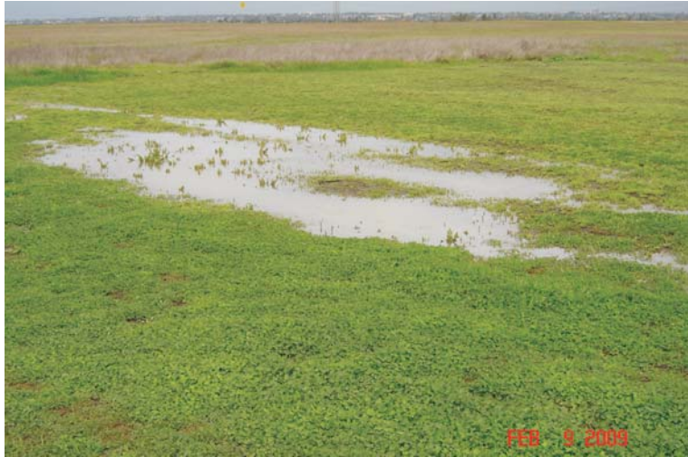
Ponding clearly evident in shallow depression at Fairview Park.
